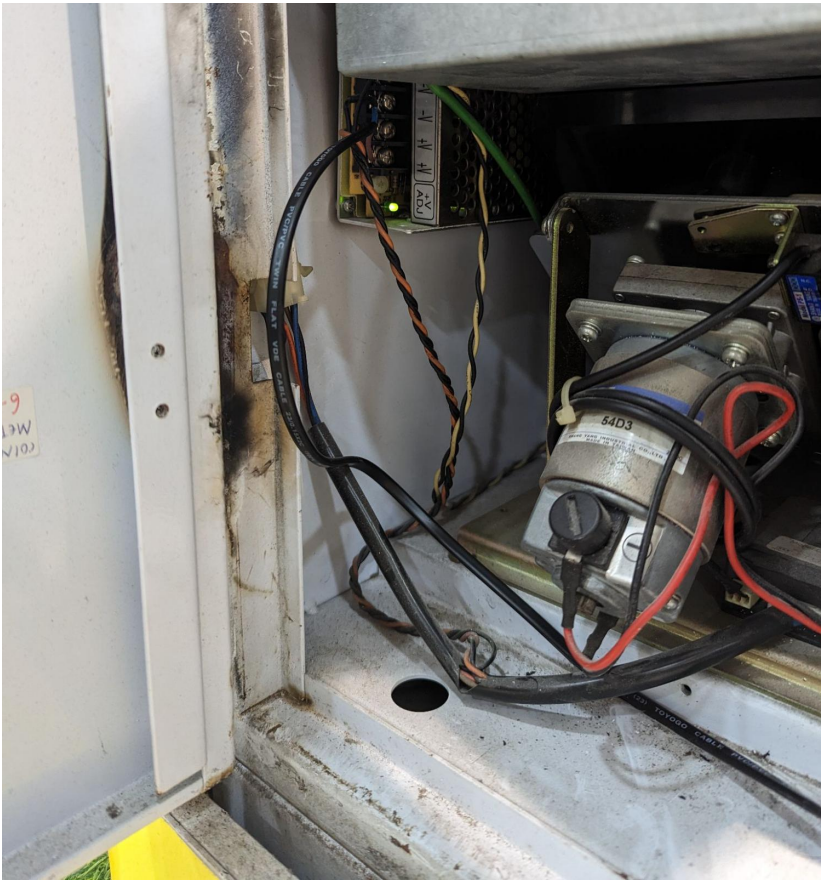
Example: Power Supply 12v connection
